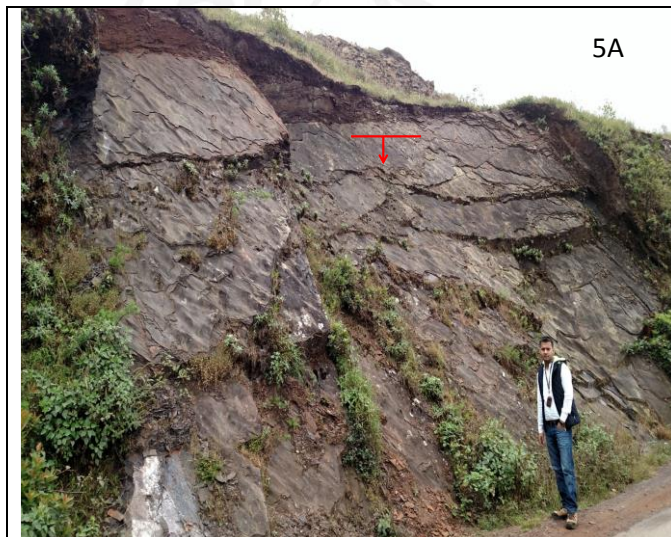
Photo 5A: Shallow Planar failure in BIF near Kavikalgundi Village
