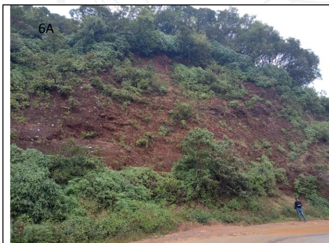
Photo 6A: Shallow Debris Slide on Weathered BIF on Attigudi- Bababuda Road section
