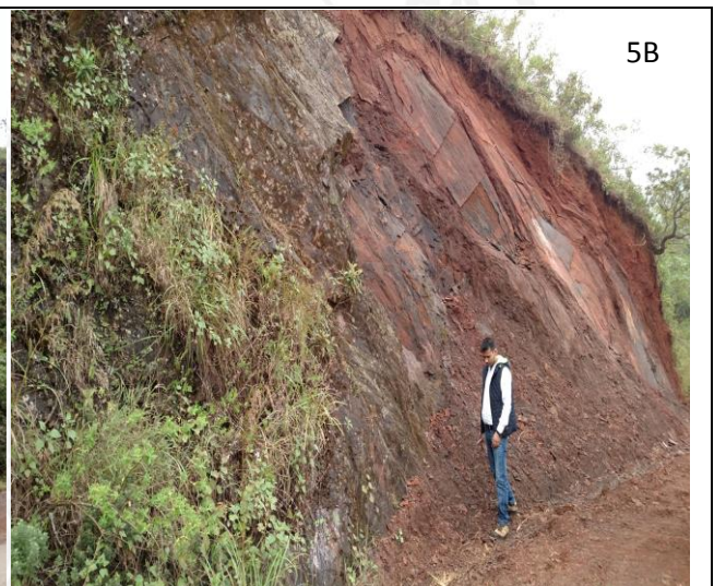
Photo 5B :Shallow Planar failure in BIF near Kavikalgundi Village
